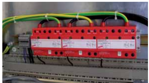
Fig. 9.16.4 Application of DEHNbloc Maxi coordinated lightning current arrester for 400/690 V TN-C systems
