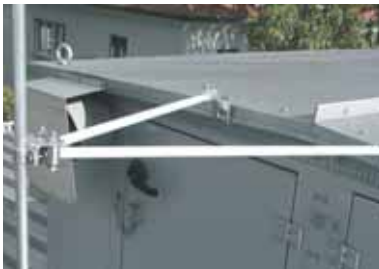
Fig. 5.1.8.4 Angled support for air-termination rods
