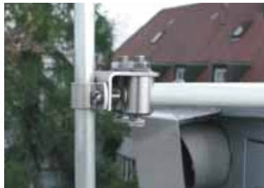
Fig. 5.1.8.5 Supporting element for the air-termination rod
