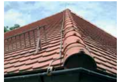
Fig. 5.2.2.1.3 Air-termination system with connection to the gutter
