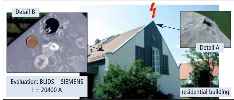
Fig. 5.1.4.2 Example of damage: Metal plate cover
