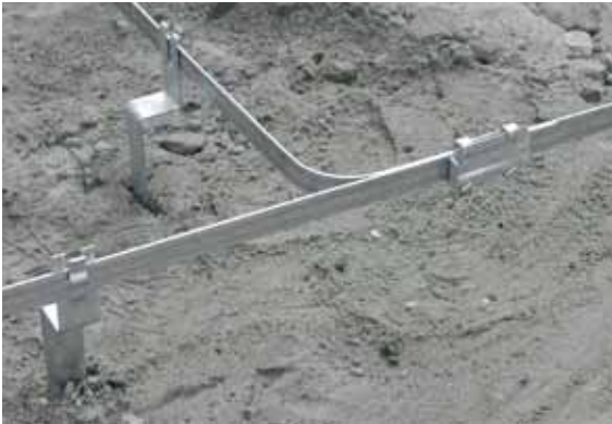
Fig. 5.5.2.3 Foundation earth electrode
