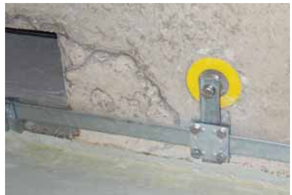
Fig. 7.7.1.1 Ring equipotential bonding and fixed earthing point for connection of metal installations
