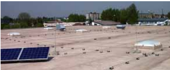
Fig. 5.1.3.3 Use of air-termination rods
