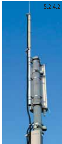
Fig. 5.2.4.1 Isolated air-termination system with distance holder Fig. 5.2.4.2 Isolated air-termination system for cell sites – Application of DEHNconductor system
