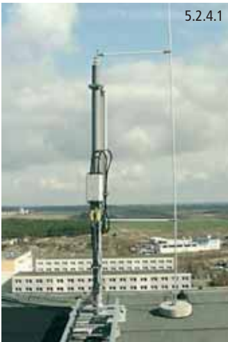
Fig. 5.2.4.1 Isolated air-termination system with distance holder Fig. 5.2.4.2 Isolated air-termination system for cell sites – Application of DEHNconductor system
