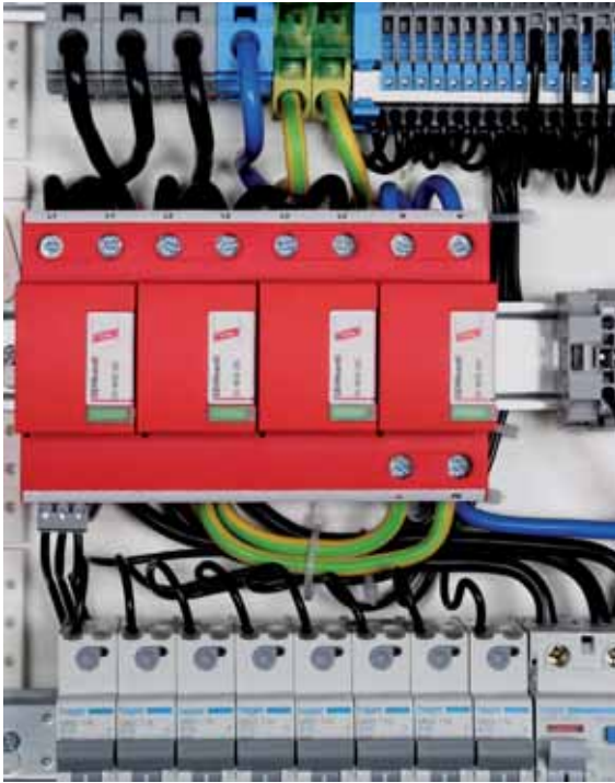
Fig. 7.5.2.5 DEHNventil combined lightning current and surge arrester
