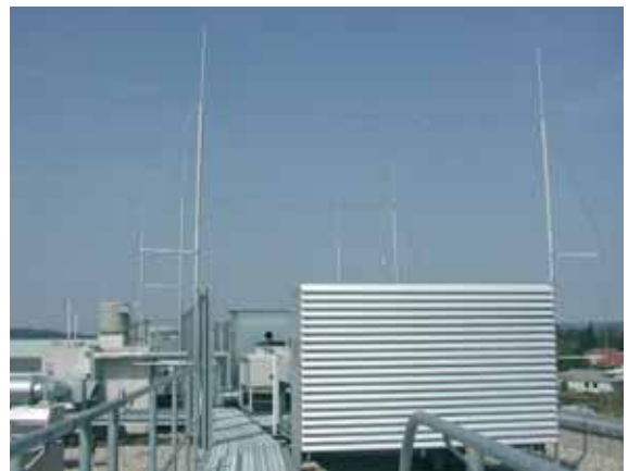
Fig. 5.1.8.12 Isolated air-termination systems with DEHNiso-Combi
