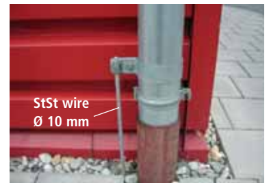
Fig. 5.2.2.1.4 Earthed downpipe
