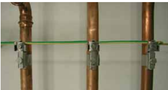
Fig. 6.1.6 Equipotential bonding with straight-through connection
