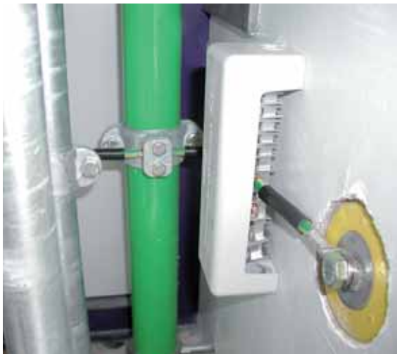
Fig. 7.5.1.1 Connection of EBB with fixed earthing point
