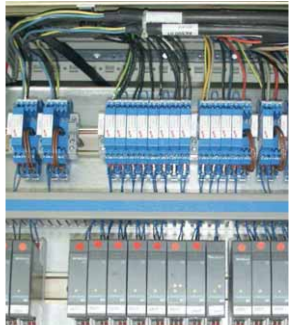
Fig. 9.15.6 BCT MOD MD EX 24 for intrinsically safe circuits
