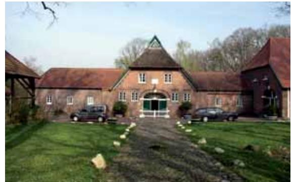
Fig. 5.1.5.4 Historical farmhouse with external lightning protection (Ref. Photo: Hans Thormählen GmbH & Co.KG)
