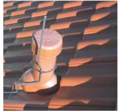
Fig. 5.1.2.3 Additional air-termination system for ventilation pipes
