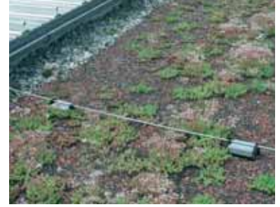
Fig. 5.1.7.3 Conductor leading on the covering layer
