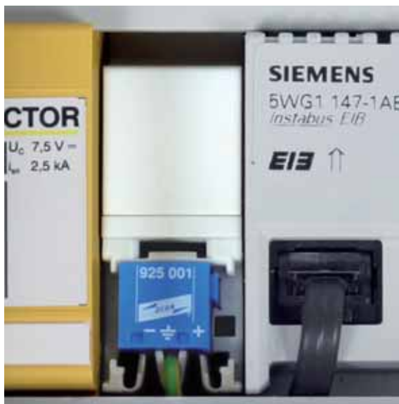
Fig. 9.10.1 Application of the BUStector (Part No. 925 001)
