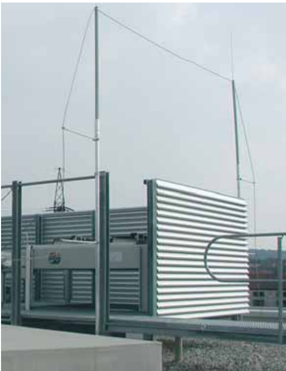
Fig. 5.1.8.14 Isolated air-termination system with DEHNiso-Combi
