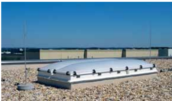
Fig. 5.1.1.17 Protection of small-sized installations on roofs against direct lightning strikes by means of air-termination rods
