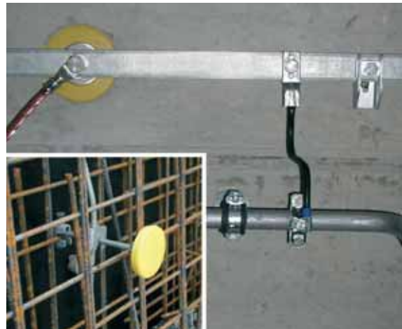
Fig. 5.5.2.8 Fixed earthing terminal
