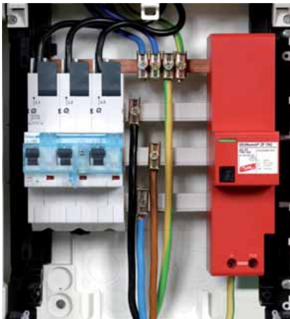
Fig. 6.2.2 DEHNventil ZP combined arrester directly snapped on the busbars in the terminal field of the meter cabinet
