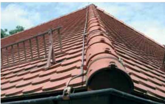
Fig. 5.1.1.18 Gable roof with conductor holder
