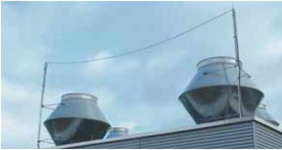
Fig. 5.2.4.2.3a Fan with air-termination rod and spanned cable
