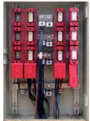
Fig. 8.1.6.6 Surge protective device Type 2 V NH for use in NH fuse bases
