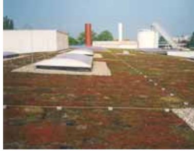
Fig. 5.1.7.2 Air-termination system on a green roof
