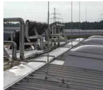
Fig. 5.1.4.7 Air-termination rod for a dome-light on a roof with round standing seam
