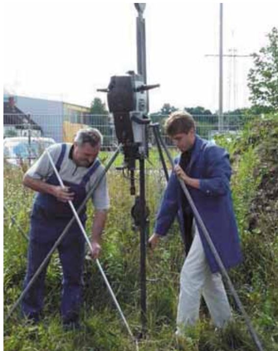
Fig. 5.5.4.2 Driving the earth rod in with a work scaffolding and a vibrating hammer
